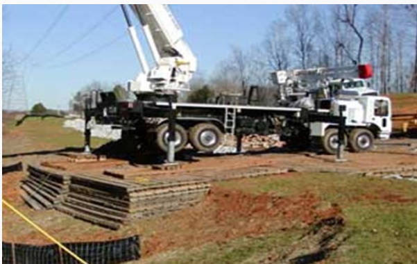
Utility Vehicles and Man lift chassis
